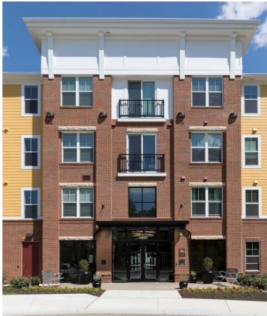
Coan Pond Residences; Fairfax, VA. Photo courtesy of Residences at Government Center.
